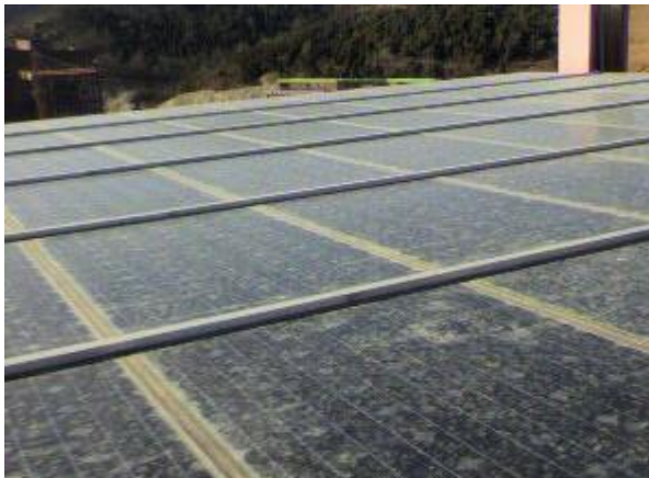
Solar panel with yellow sand accumulation
