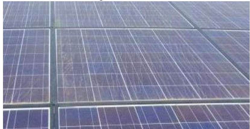
Solar panel on which yellow sand accumulated again after cleaning water had dried out
