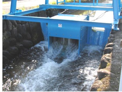
Small Hydro Stream EV plug-in station
