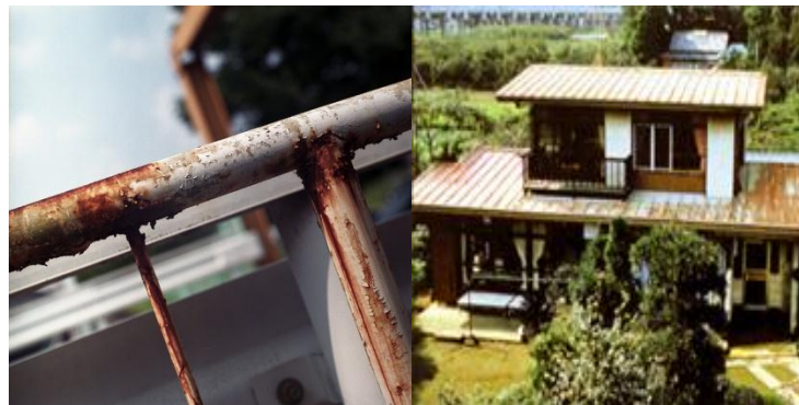
handrail and house
