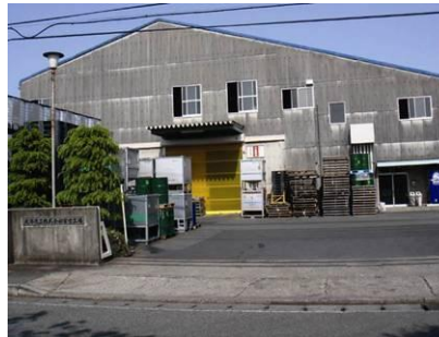
Fuji Factory (Fuji-shi) KR bonding
