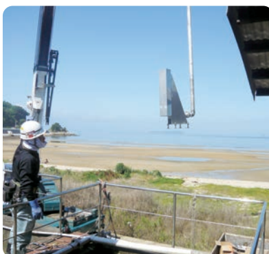
KUH KAI installation condition
