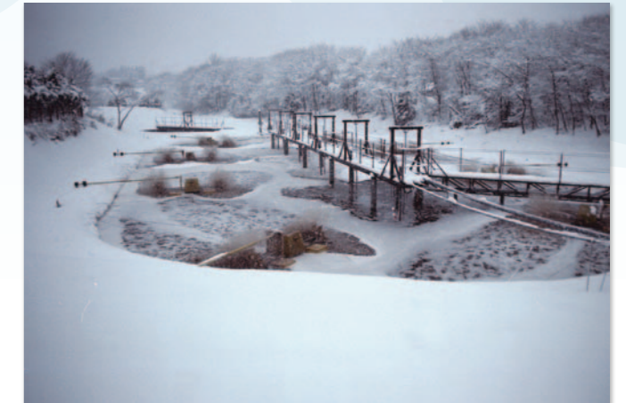
Advanced Treatment Plant for Domestic Wastewater (Air Temperature - 15°C / Water Temperature 0°C) 90% nitrogen removal / MLSS 5000mg/l
