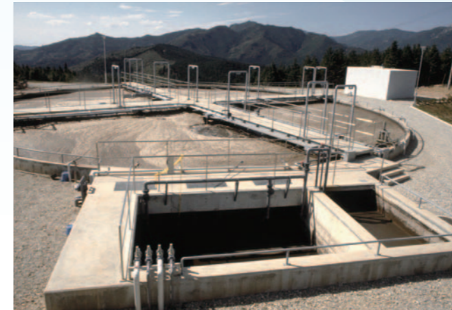
Advanced Treatment Plant for Domestic Wastewater (not categorised by Former Ministry of Health & Welfare) 30m diameter / 8m water depth / effective capacity 3000 m 3
